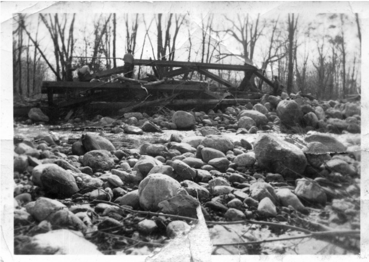
Wooden truss in Hartland Hollow Bridge.
