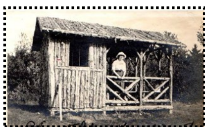
1915 photo of cabin on Foster’s pond
